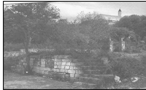
Foundation of Old Parham School, 2007
