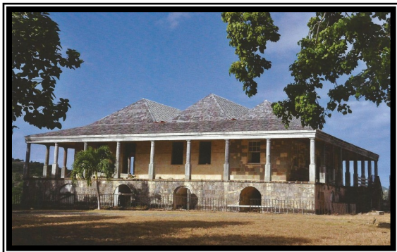
Clarence House during restoration process
